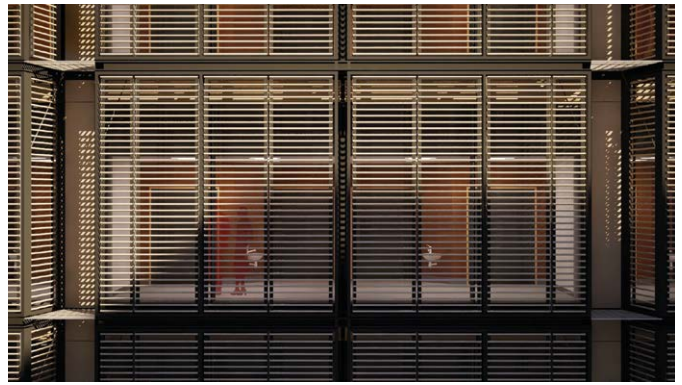
An adjustable venetian blind system is incorporated as a non-integral part of the curtain wall system.
