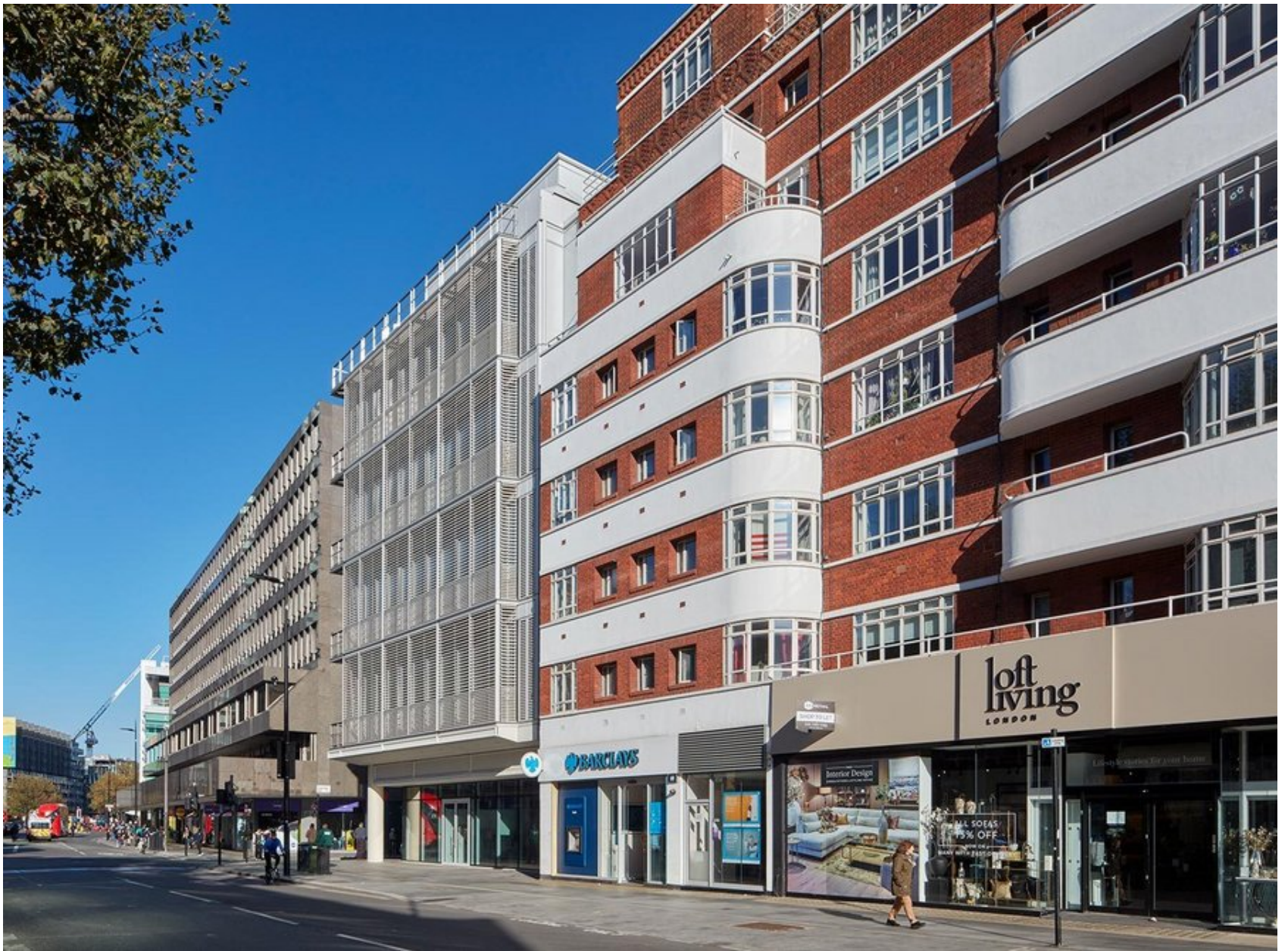
North-west corner of the building on the corner of Tottenham Court Road and Grafton Way. Credit: Paul Raftery
