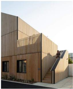
**Edward Williams Architects** demonstrated that it was less viable: the size of the structural elements, slabs and walls would increase significantly. Ultimately, they were able to prove that timber was the most efficient option.
