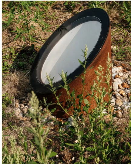
Circular skylights punctuate the wildflower roof | Credit: Fred Howarth
