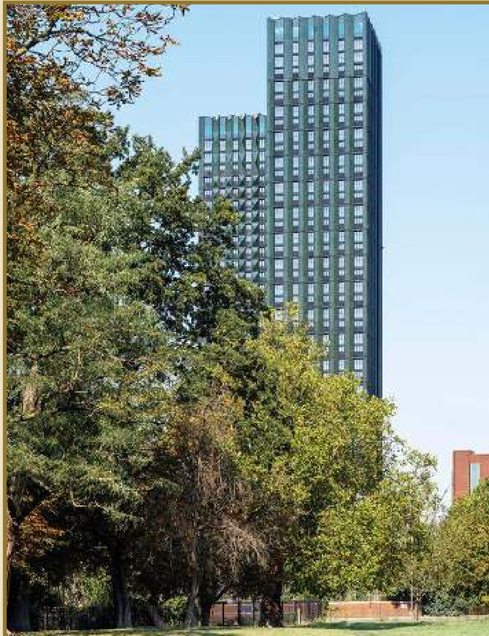
Ten Degrees in the LB Croydon by HTA and Tide Construction is the world’s tallest modular building delivered in just 26 months using modern methods of construction, completed in 2020. © HTA Design LLP
