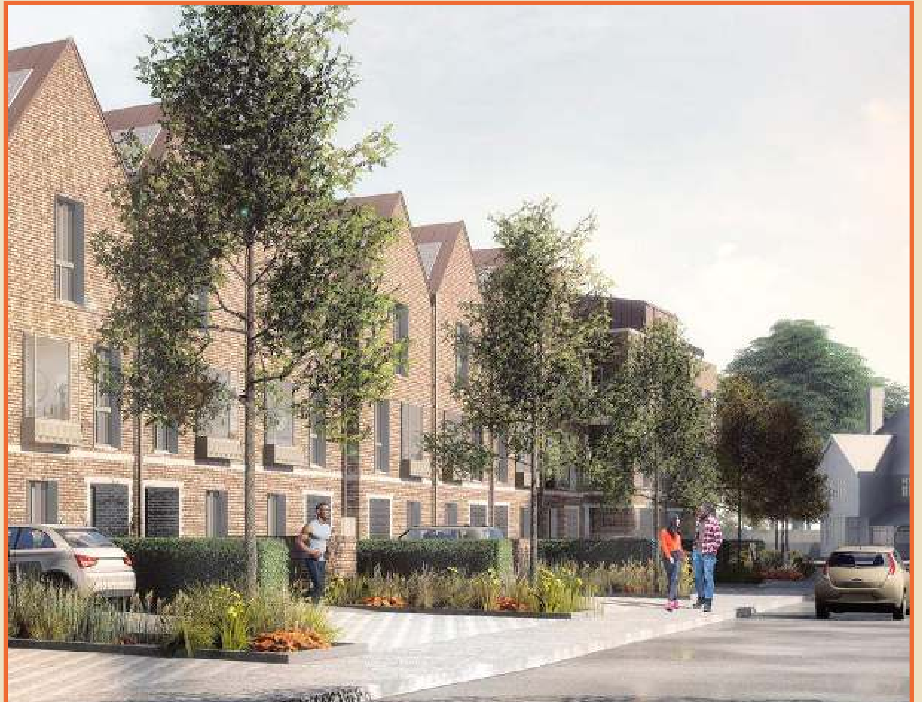
Merton Regeneration - Ravensbury by HTA Design in the LB Merton is one of three estates that Clarion are regenerating within the Merton Regeneration Project, located alongside the Wandle the masterplan reconnects the estate to its parkland setting. Completion in 2025.
