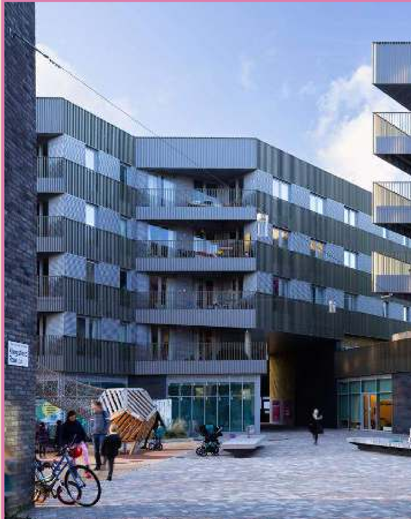
East Wick + Sweetwater by Studio Egret West, astudio London and Places for People in the LB Hackney and is the first phase of a new neighbourhood in Queen Elizabeth Olympic Park has been completed in 2021, providing the area with 302 homes, a nursery and a Co-op branch. © Chris Hopkinson, Chromaphotography
