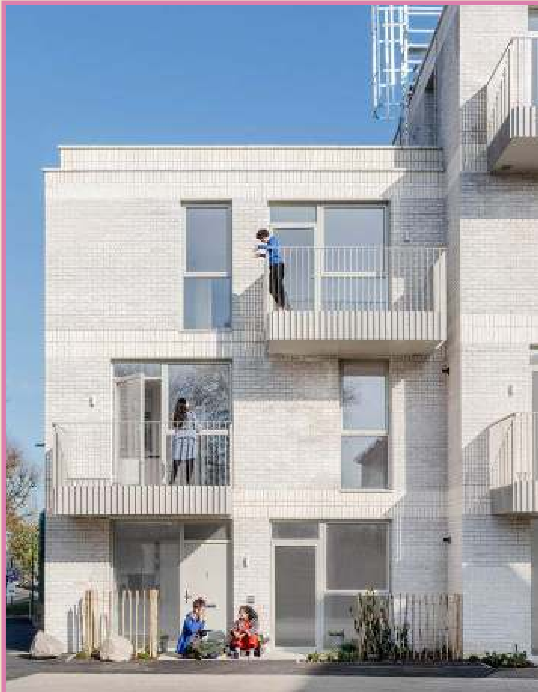
Citizens House is the first community land trust in London that has been directly created by the community using London CLT's unique affordability model, in partnership with Lewisham Citizens, Lewisham Council and the Greater London Authority. Completed in 2023 © French+Tye
