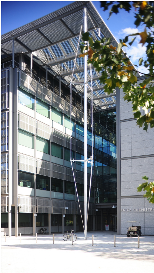
The Frick Chemistry Laboratory Building, Princeton University, USA
