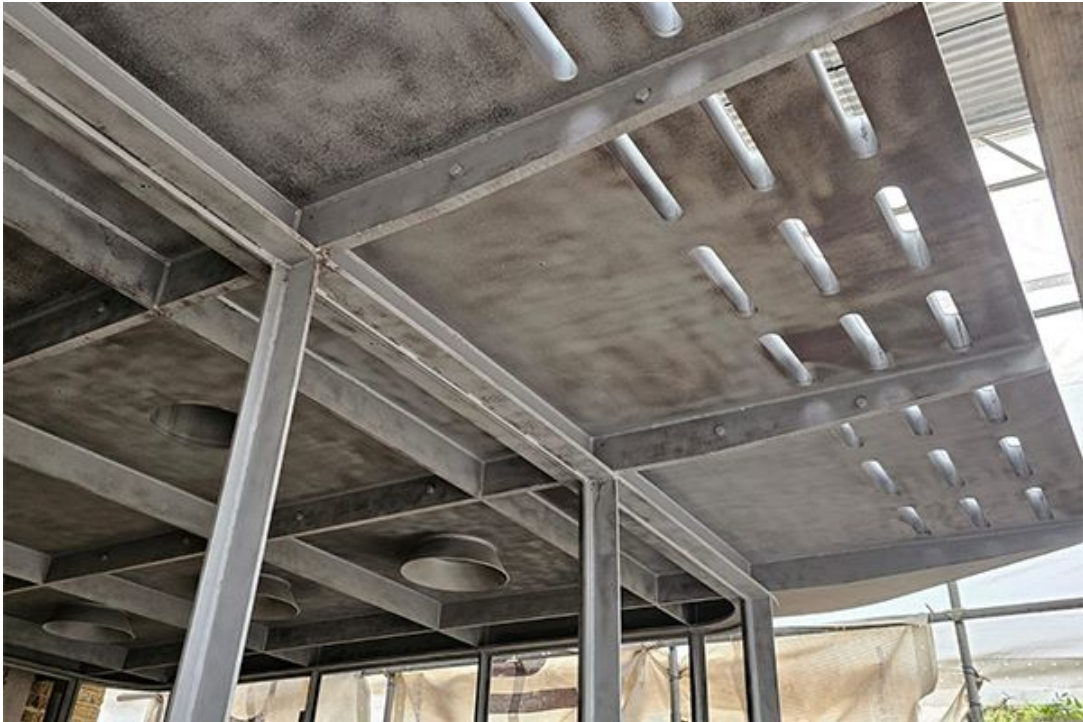
The new gallery roof after the grit blasting process.
