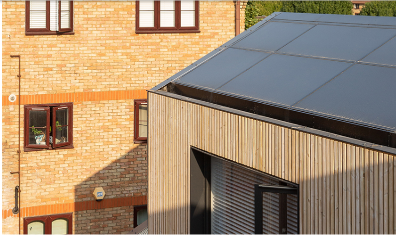
The edge to edge PV glass roofs against the existing buildings
