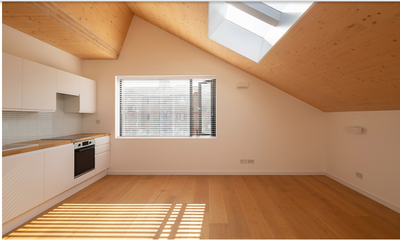
All interior ceilings are the exposed timber structure
