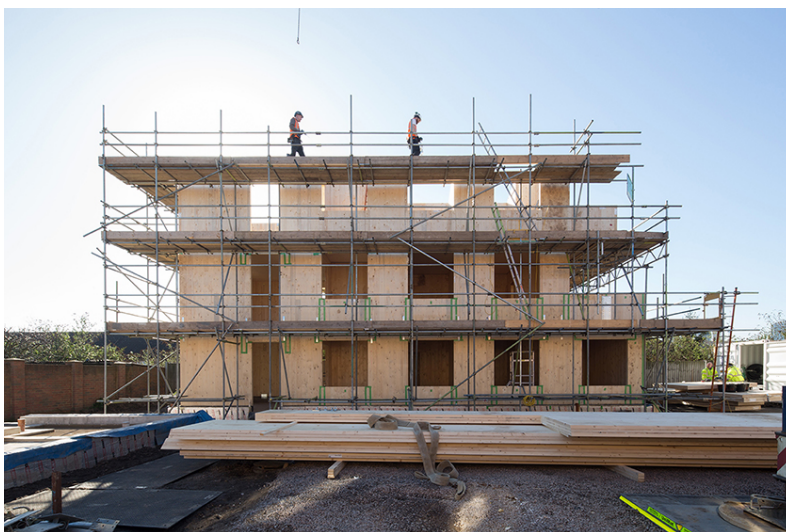
Timber structure under construction
