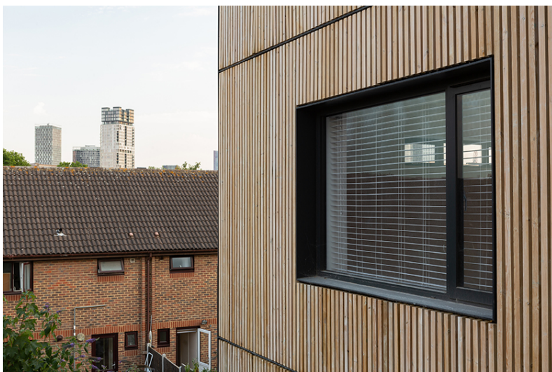
The hit and miss timber facades with the aluminium window surrounds and floor markers
