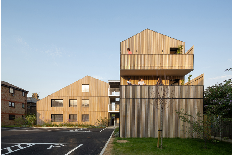
Dawn view of the East Courtyard buildings
