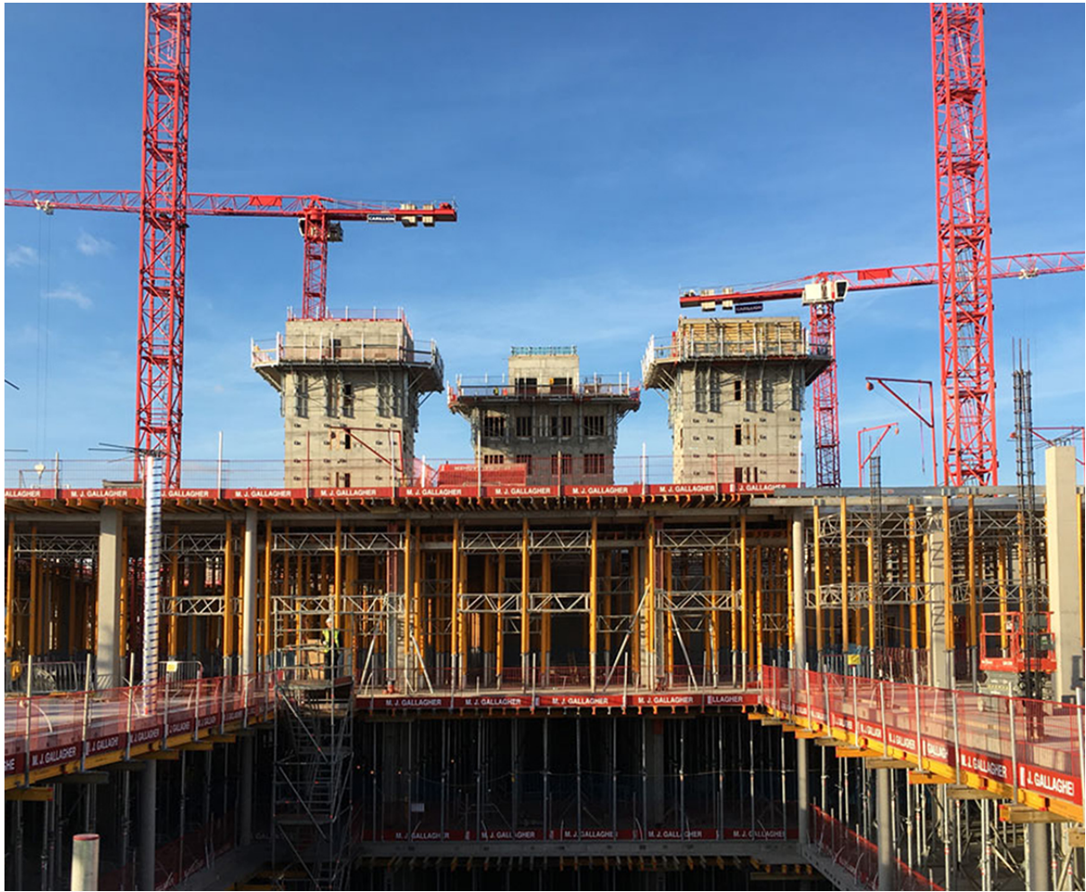
The Midland Metropolitan Hospital construction site in Sandwell, Birmingham, UK
