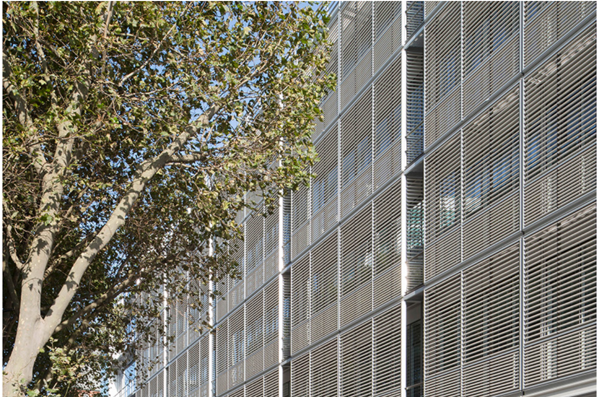
Detail of the University College London Grafton Way Building facade
