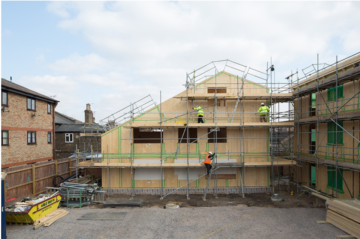
Cross Laminated Timber structure (mass timber) being installed on site
