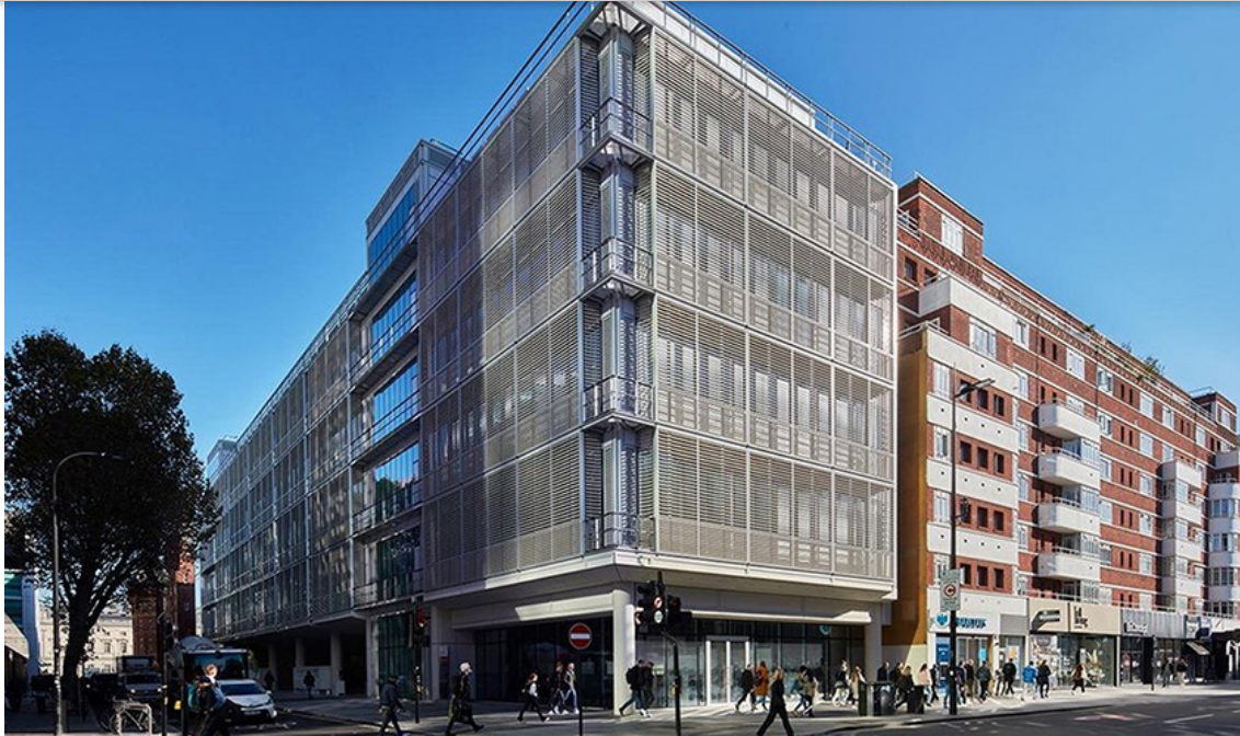
The Grafton Way building, London, UK
