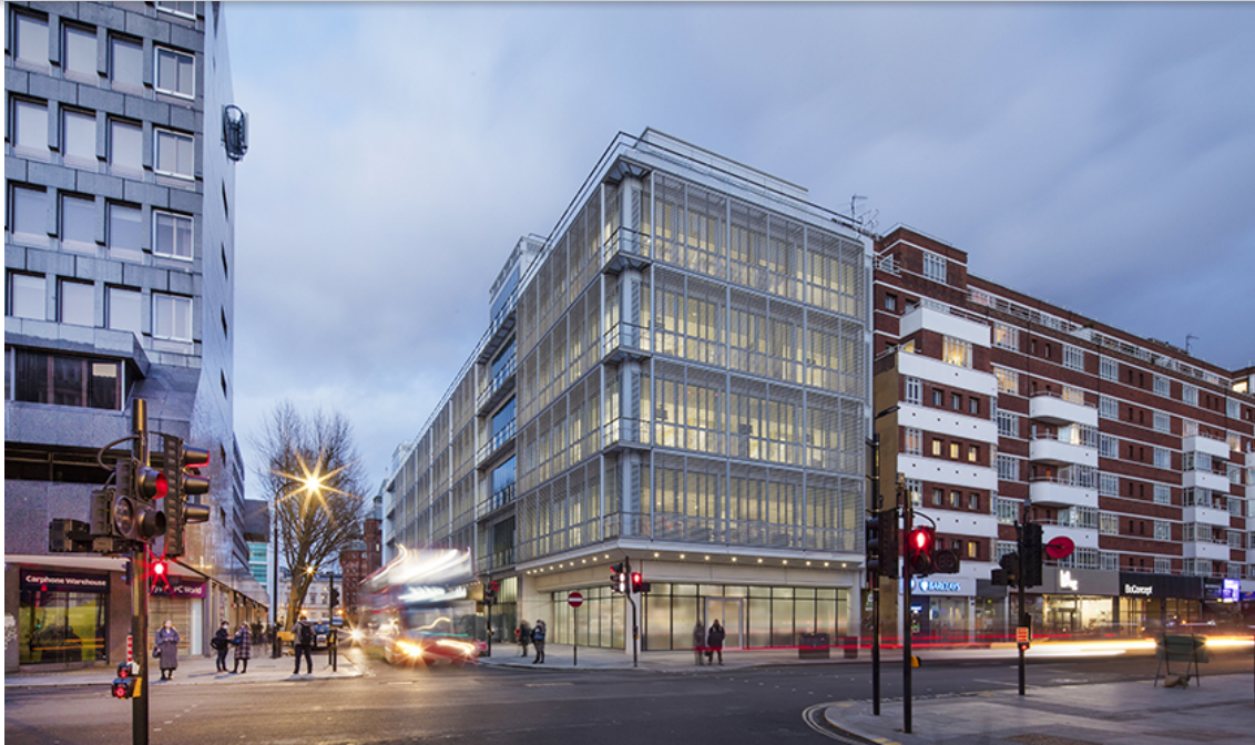
The Grafton Way UCLH building photographed from Tottenham Court Road, London.
