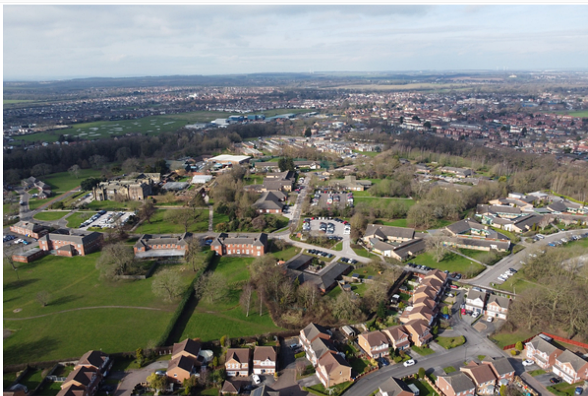
Doncaster Tickhill Road mental health NHS campus where we are implementing an ambient loop
