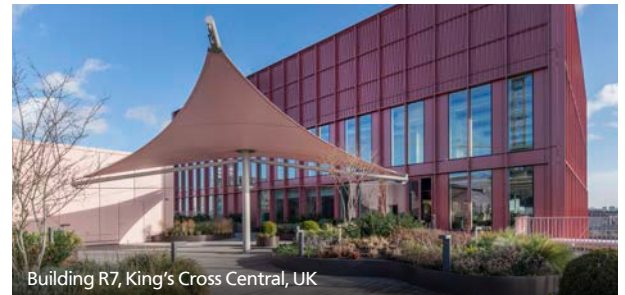
Building R7, King's Cross Central, UK
