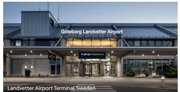
Landvetter Airport Terminal, Sweden
