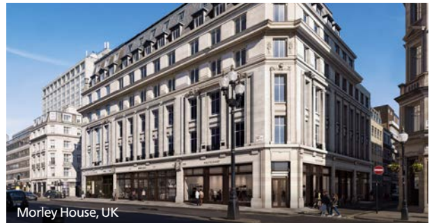
Morley House, UK
