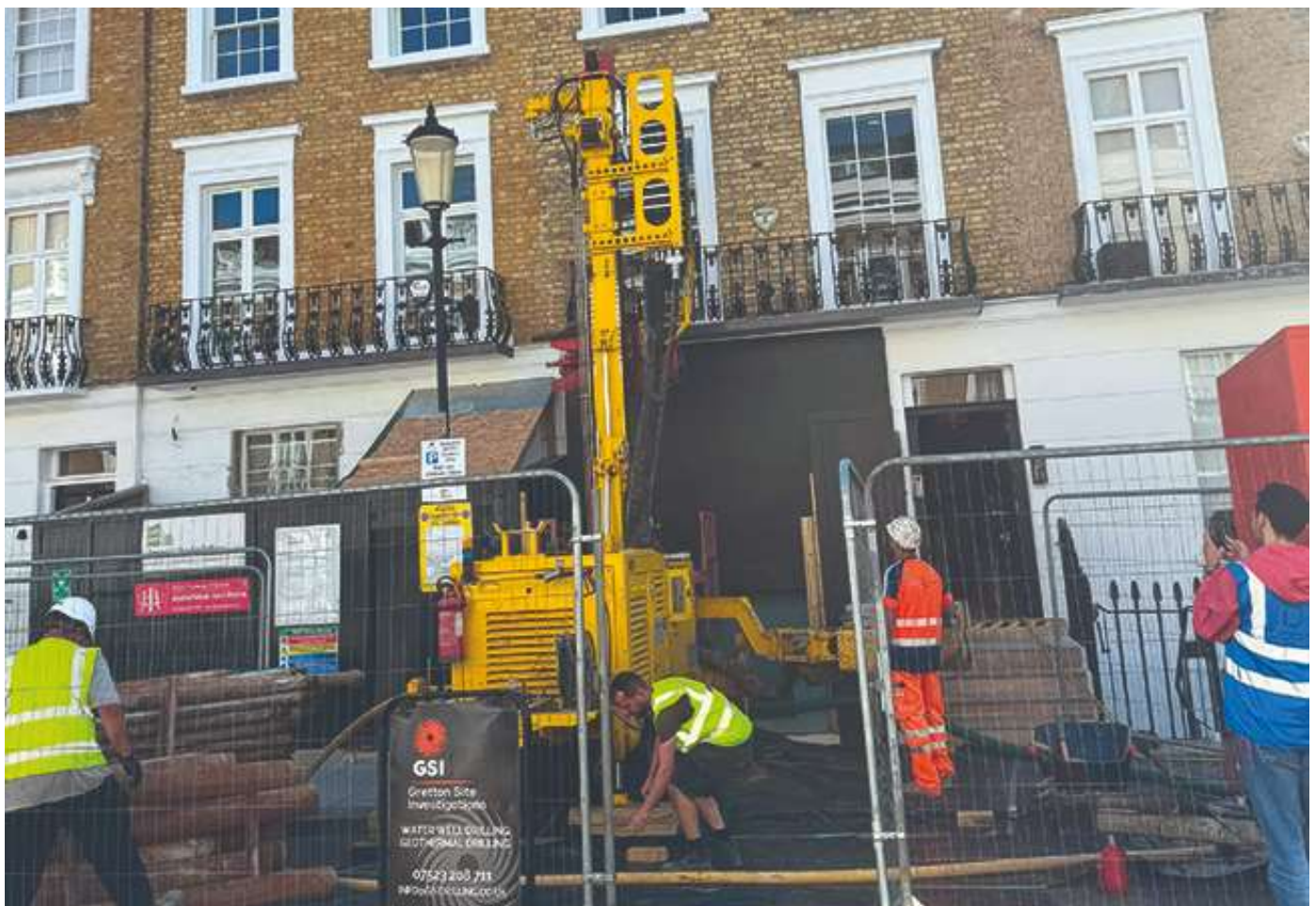
Two boreholes were drilled in the curtilage of the terraced home
