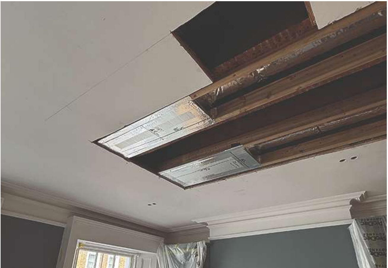
Integrating ductwork into the historic townhouse demanded close cooperation between the engineers and architects
