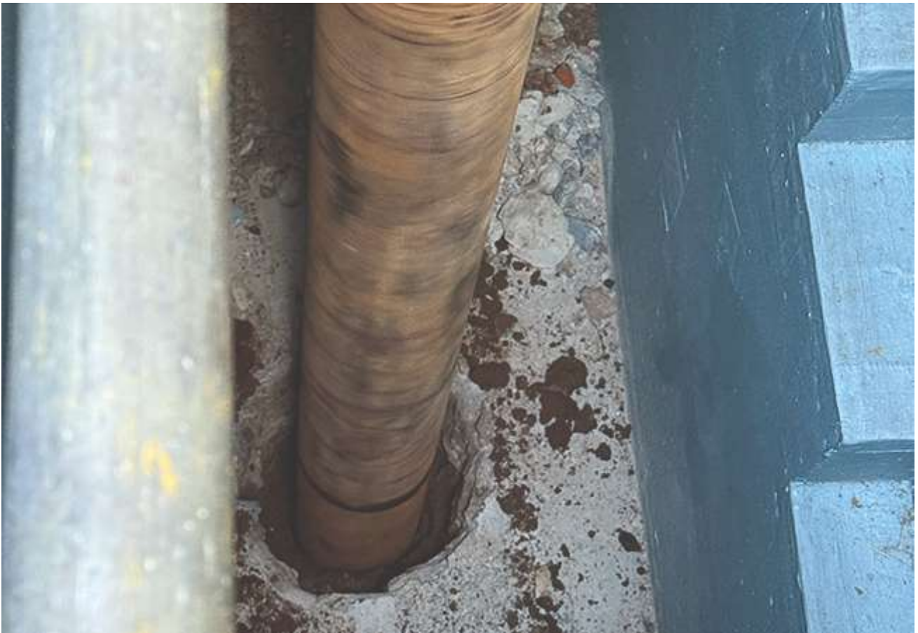
The borehole next to the property's front steps
